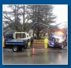
Figure 1: Using the District's vacuum truck to excavate a 6-inch diameter hole for a 20-foot deep groundwater monitoring well. This well is at the intersection of Maquoit Road and Mere Point Road.
