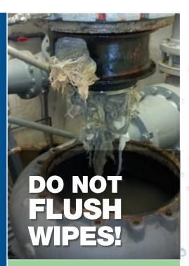
Do you think that flushable wipes are really flushable? Think again. Pictured here is the result of wipes entering our wastewater system and plugging a pump. The "flushable" wipes do not break apart like toilet tissue. The fiber in the wipes are so strong that they collect in the pumps and plug them. They create a costly maintenance nightmare, and an environmental hazard if it causes an overflow in our system.
